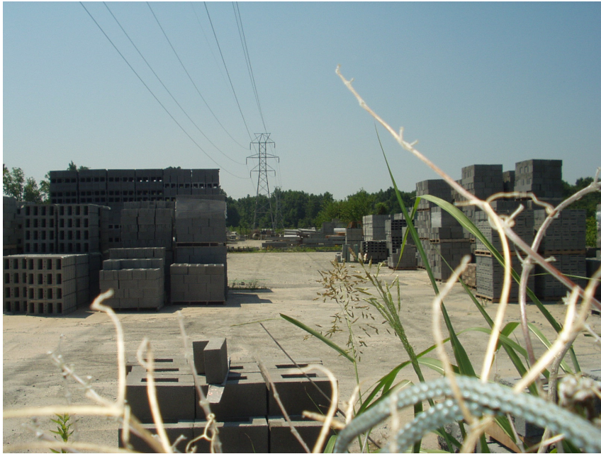
Photograph 1 – View from south to north along Johnson Concrete / FCX property line.
